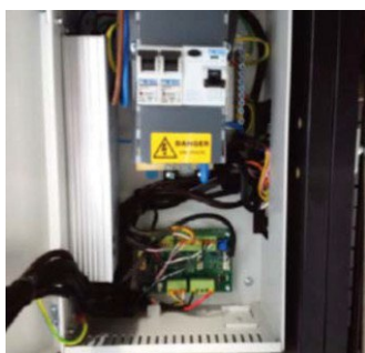
4. Control box open showing main PCB
