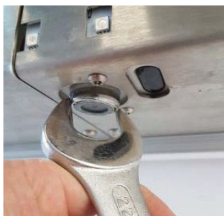
2. Use a 22mm spanner to turn the aerator counter-clockwise (anti-clockwise to undo)
