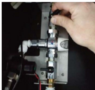
1. Isolate the water supply locally
