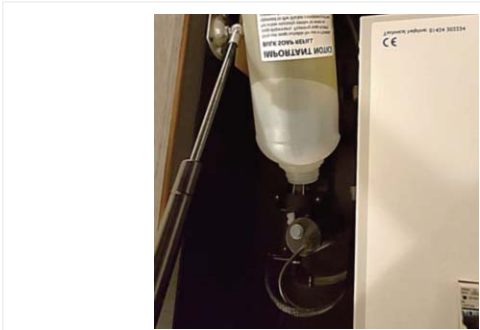
3. Unscrew the soap tank from the pump housing and lower out, refill and replace
