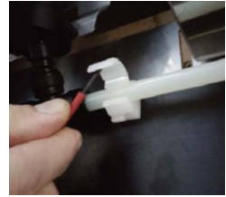
3. Open the pipe clips at the tee
