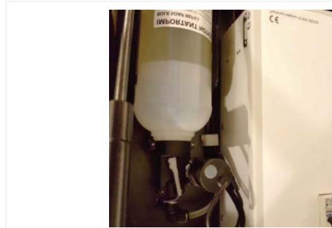
4. Prime pump by locating and depressing the grey button on the pump housing as indicated here until soap flows
