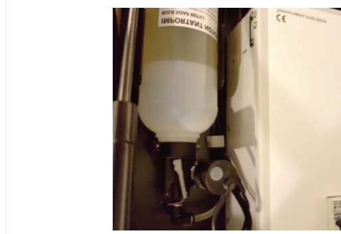
2. The soap tank with grey override button on pump housing indicated
